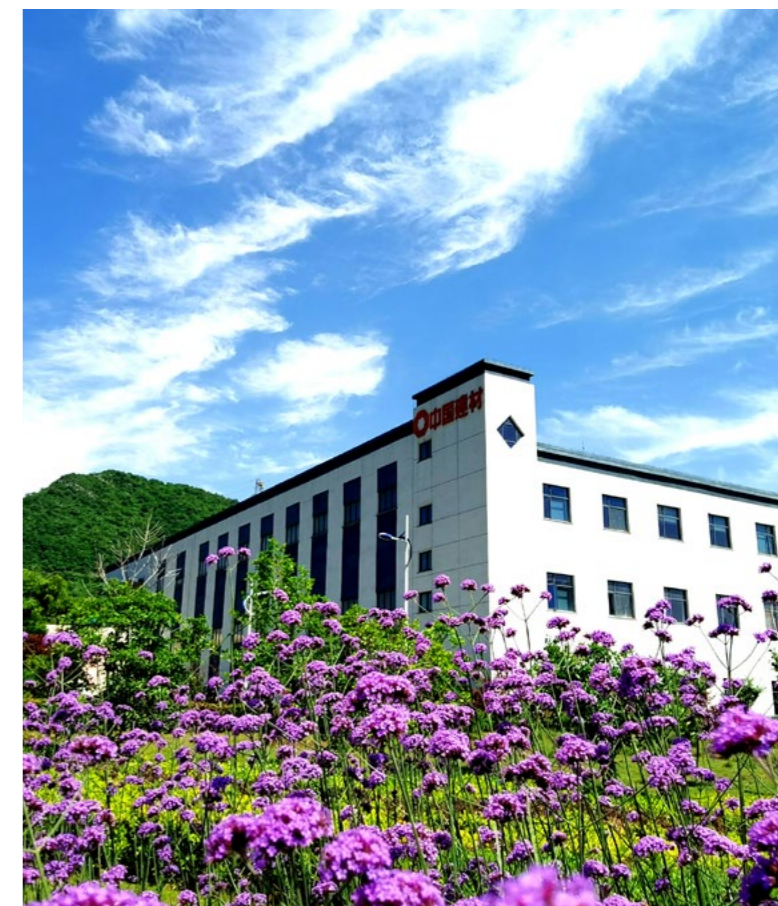
Production Workshop for Co-disposal of Domestic Waste in Cement Kilns of Sinoma Anhui
