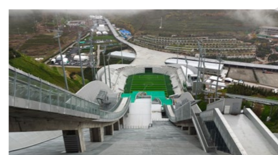
China Building Materials Academy (CBMA) ensures safety for Winter Olympics with environmental governance technology
