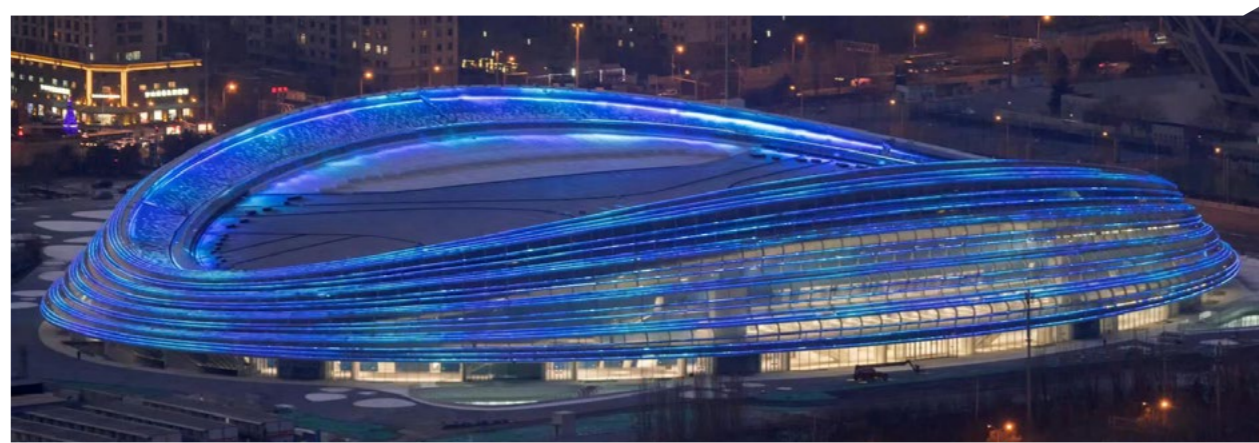
National Speed Skating Oval (also called "Ice Ribbon") uses 80,000 square meters of BNBM plasterboards and 70 tons of "Dragon Brand" light steel-frame structures
