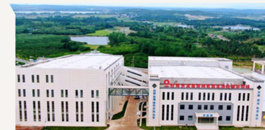
Project of co-disposal of 500t/d domestic waste using cement kilns of Jiangsu Hantian Cement Co., Ltd.
