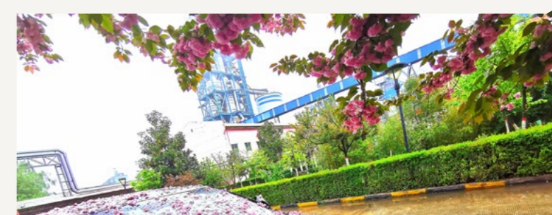
A panoramic view of Chengxian Qilianshan Cement Co., Ltd.
