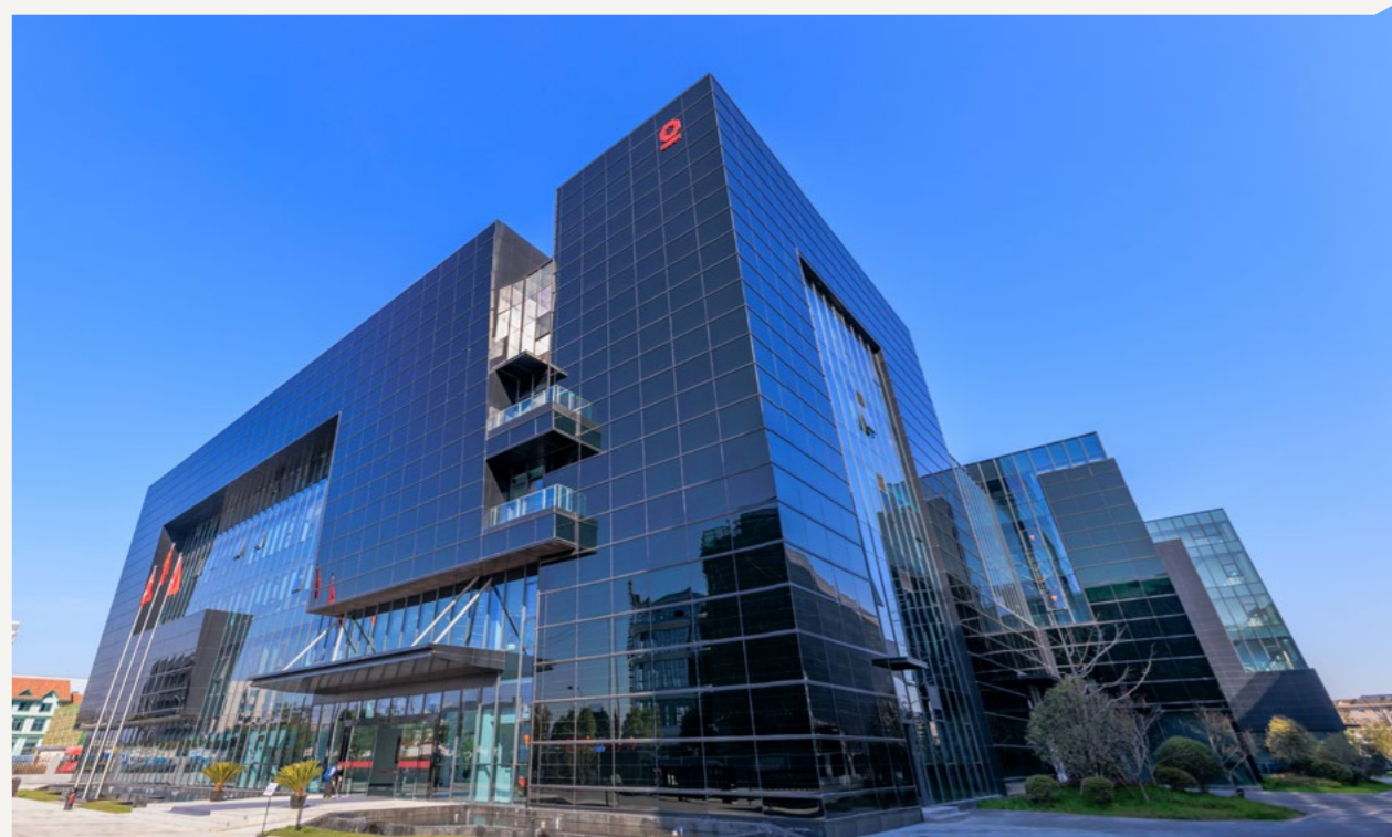
China's first CdTe power generation glass integrated project in a city center -- Shanghai Songjiang Triumph Robot Building
