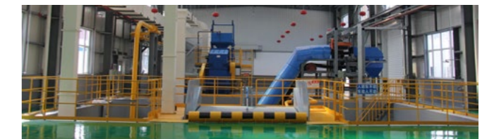
Nanjing CUCC Hazardous Waste Disposal Workshop
