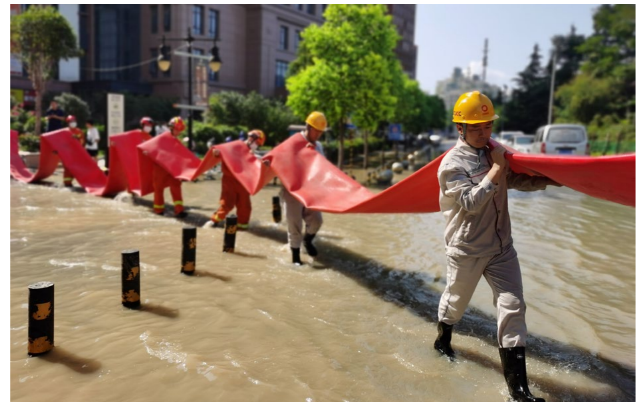
▼ Pioneer Commando consisting of the Party members in China United Cement Dengfeng Co., Ltd participated in the laying of drainage pipeline at the rescue point.
