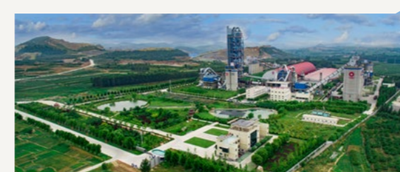
A panoramic view of Green Intelligent Factory of China United Cement Tai'an
