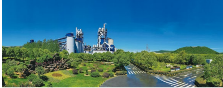
▼ Huaikan Nanfang Intelligent Cement Factory
