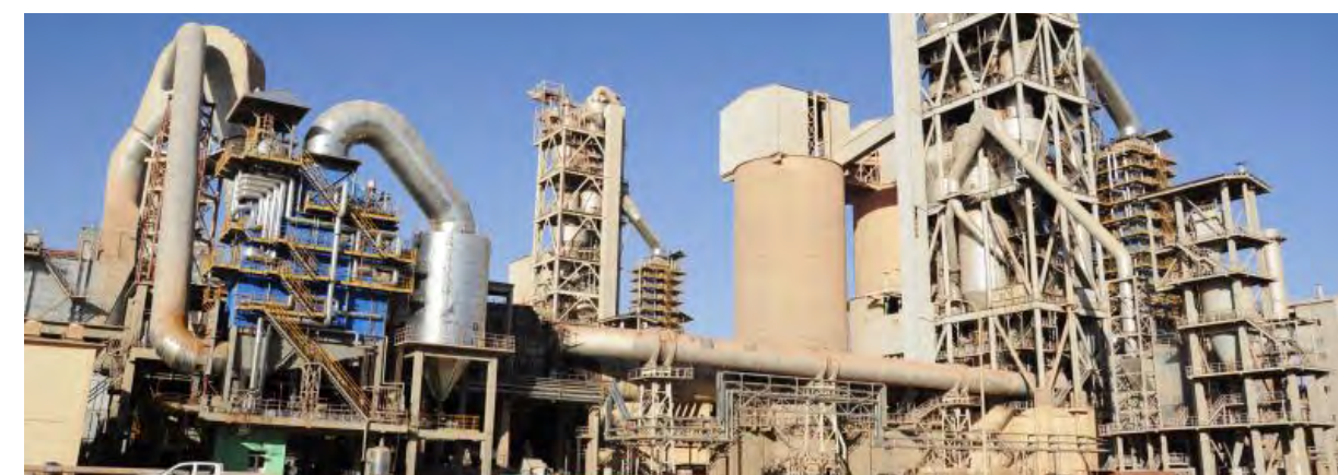
YCC Waste Heat Power Generation Project in Saudi Arabia
