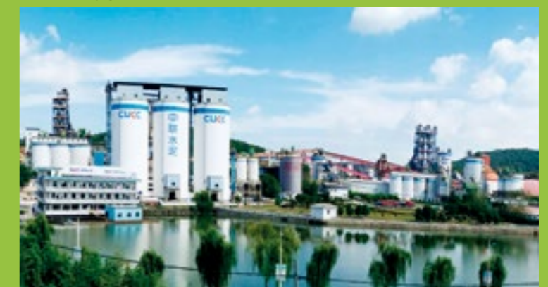
A full view of the 3 Million m 3 /y Technological Transformation (Relocation) Project initiated by China United Concrete Nanjing Co., Ltd.
