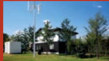
The air-suspension fan is equipped with a battery energy storage system (daily generated energy: 2 kWh).
