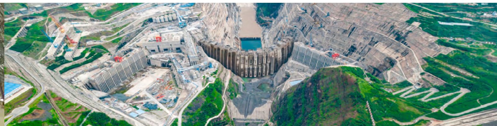
© China Building Materials Academy' Low-heat Cement Powers Baihetan Dam in Building a "Seamless Dam"
