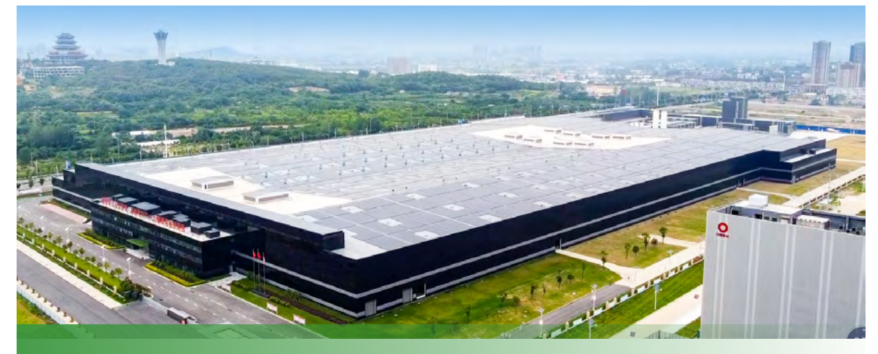
◎ Triumph Science & Technology's Stand-alone 10MW Thin-film BIPV Application Demonstration Project
