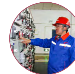
Yongdeng Qilianshan Cement Group
