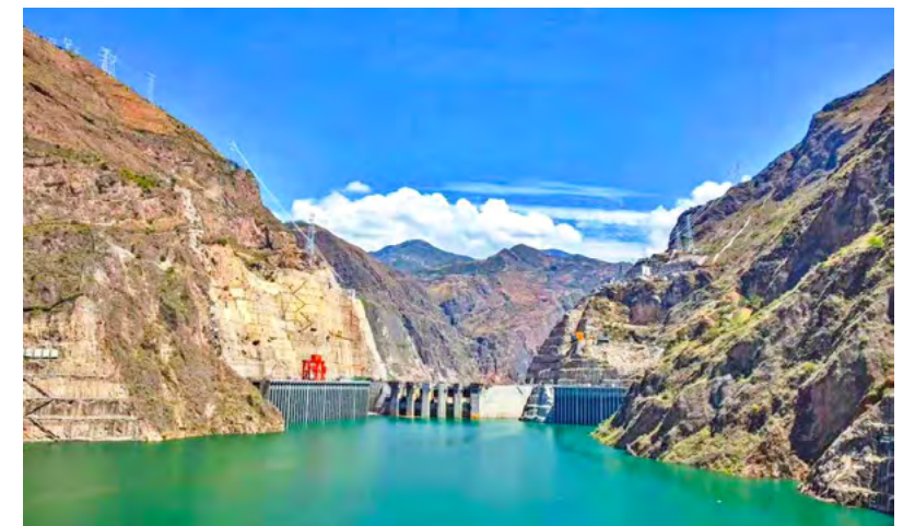
© China Building Materials Academy helps build the world's thinnest dam in Wudongde Hydropower Station with low heat cement
