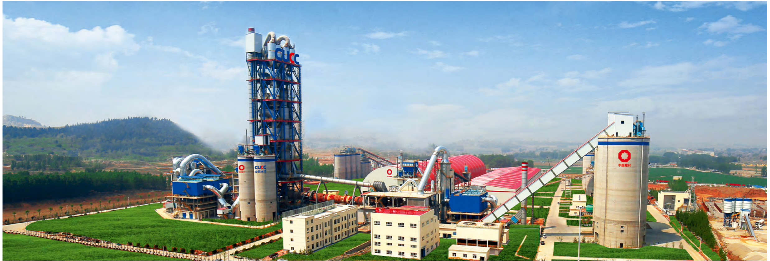
China United Cement Corporation (Tai'an) Industrial 4.0 Intelligent Cement Factory
