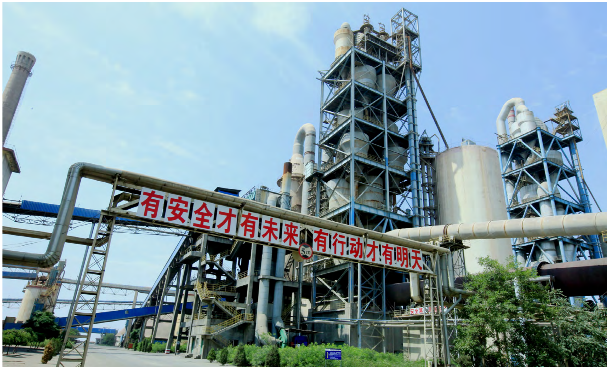
Factory of Ningxia Qingtongxia Cement Co., Ltd.
