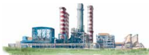
Newly-built refuse incineration power plant with a daily disposal capacity of 1,000 tons
