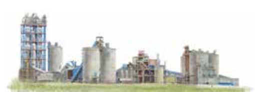
Newly-built cement plant with daily output of clinker of 5,000 tons
